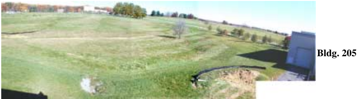
Figure 1. Initial Terrain of Construction Site.
