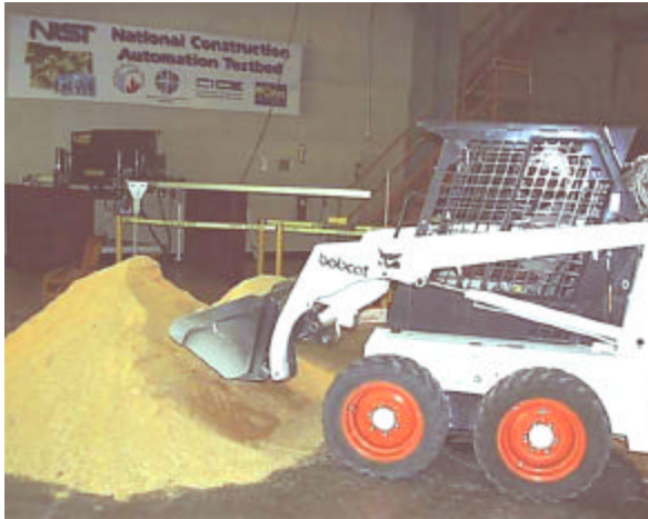
a. Sand removal.
